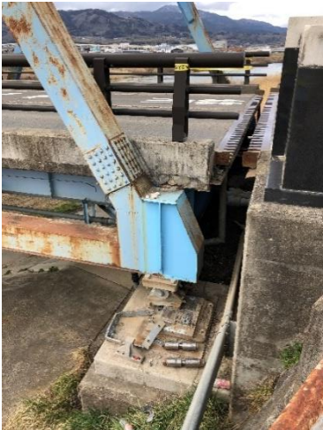
(b) East abutment
