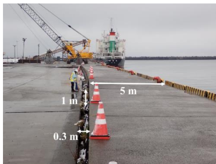
(a) Deformation at Quay No. 2
