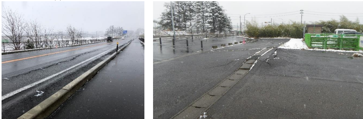
(b) Crack in Route 6 and uplift in a nearby petrol station
