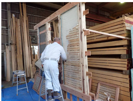
(a) Plastering on timber lath
