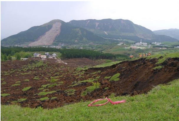
Photo 1: View of the Takanodai landslide (looking downhill), with damaged houses and the large debris avalanche at Aso Ohashi Bridge visible in the distance
