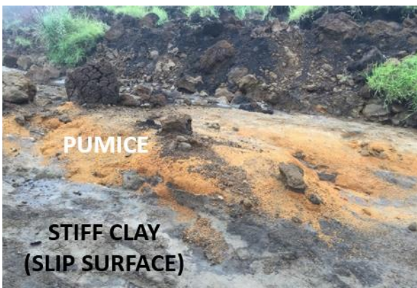
Photo 3. Traces of pumice soil on the slip surface
