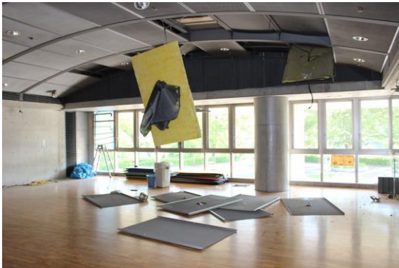
Figure 18. Ceiling failure
