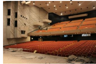
(b) After repair
