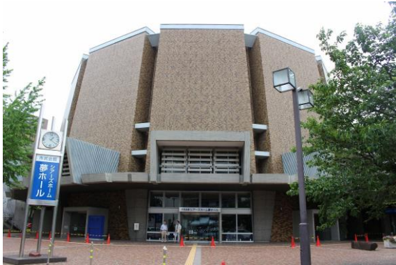
Figure 1. External view of the hall
