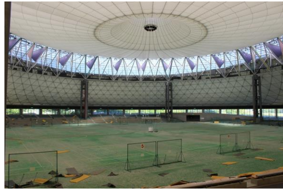
Figure 11. Internal view of the dome
