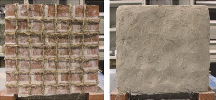
Figure 4. Photos of ARM wallet before and after plastering
