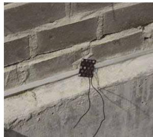
**Figure 5** Out of plane connection for PP-band
