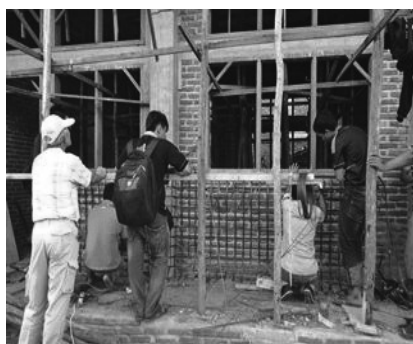
(a) PP-band retrofitting of a masonry house in Indonesia
