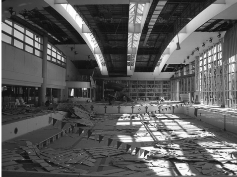
(a) Interior view of the pool
