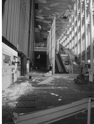
(b) The damage in the entrance hall
