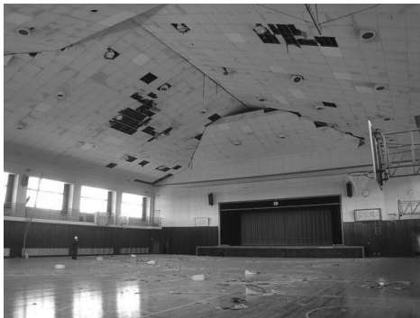
(a) Interior view of the gymnasium
