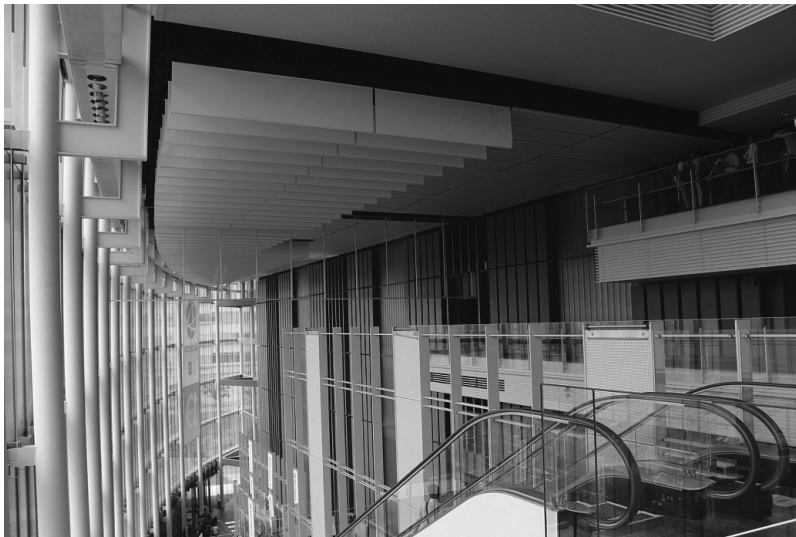
(c) New membrane ceilings
