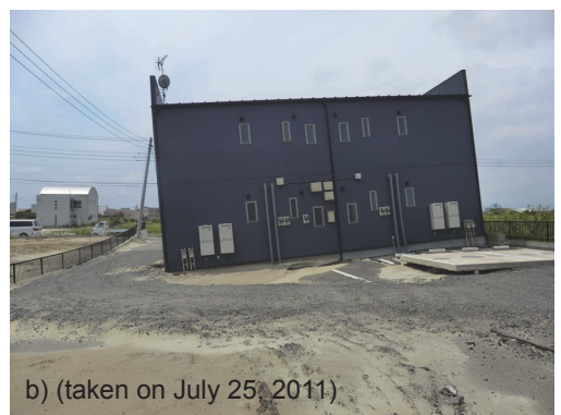
Photo 1 Sand boiling observed in a) Hinode area, Itako city and b) Fukashiba area, Kamisu city
