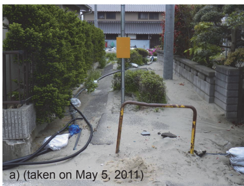
Photo 1 Sand boiling observed in a) Hinode area, Itako city and b) Fukashiba area, Kamisu city
