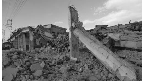
(b) Collapse of an industrial building
