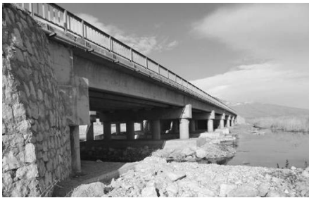
(a) Bridge with no significant damage
