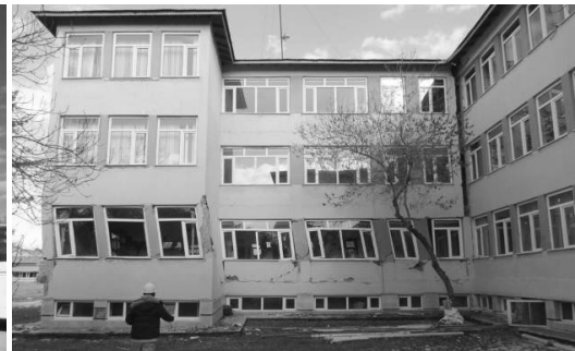
Photo 9 South side of Building C
