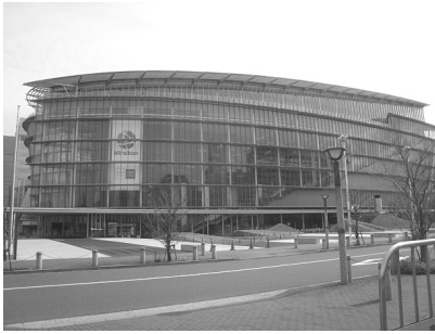
Figure 1. External view of Miraikan
