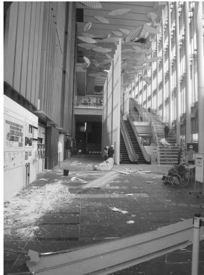
Figure 3. Internal view of the entrance hall after the disaster
