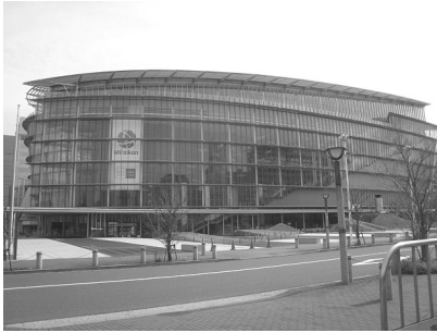
Figure 1. External view of Miraikan
