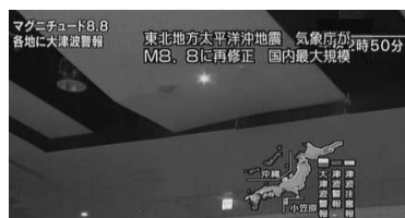
Figure 12. Ceiling just before failure (from NHK TV news)
