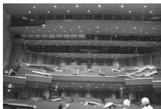
(a) Internal view
