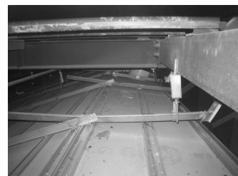
(e) Ceiling under ceiling room
