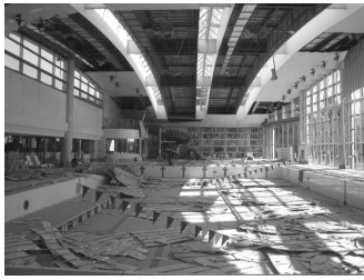
(a) Internal view
