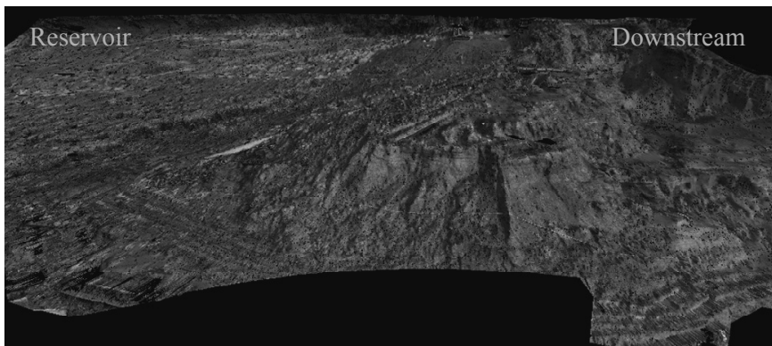
Fig. 4 3D image of the breached dam body using LPM-321
