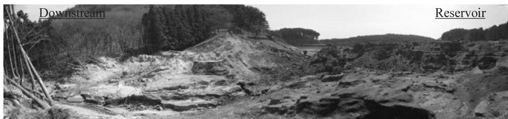
Photo 3 Breached large dam as seen from its left abutment (April 15 th at 37.302465, 140.195223)
