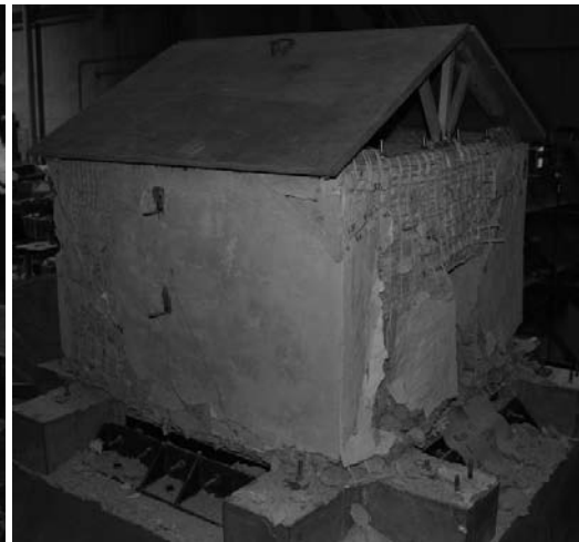
Figure 15. Retrofitted model after Run 51
