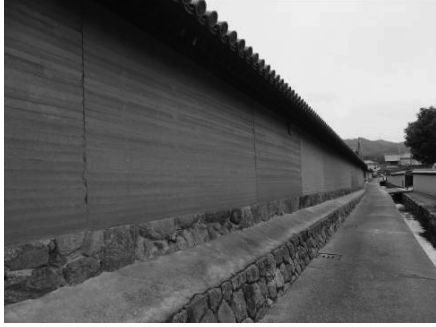
Photo 1. The rammed earth wall (“Oo-gaki”) surrounding Horyu-ji temple in Nara.
