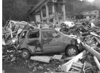
Debris piled up underneath the viaduct.
