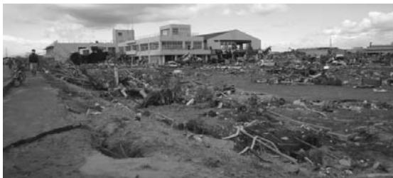
Damage to Nakano elementary school. After the earthquake, many people who had evacuated to the gym were inundated by the tsunami.
