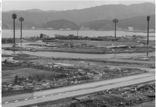
The entire city was damaged by tsunami. Takata-Matsubara-daiichi stadium was also hit.
