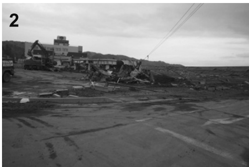
Damage to a hot spring facility
