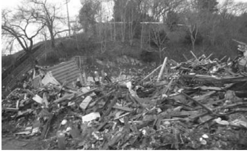
A shrine located on a small mountain was not damaged.
