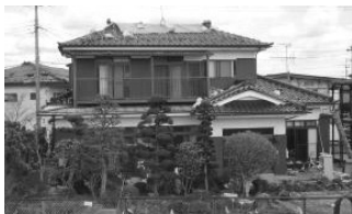
Damage to a timber house by ground motion
