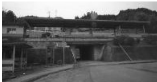
Significant damage was not seen in Sanriku station where the Okirai school students evacuated.
