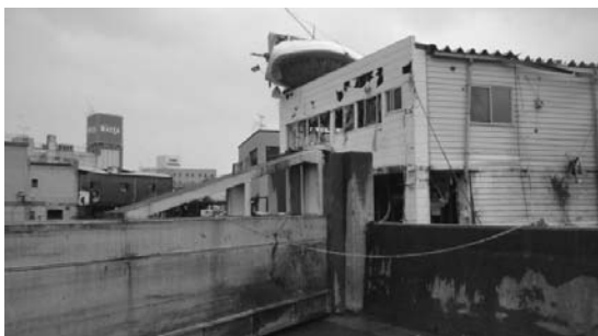
A boat was lifted up to the roof of a two-story building by the tsunami.
