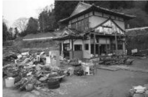
The tsunami reached the first floor of the house next to the gas station.
