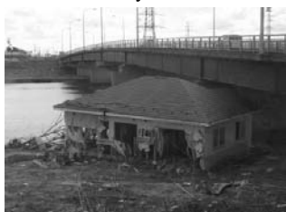
A house trapped by a bridge located about 2.5 kilometers from the coast
