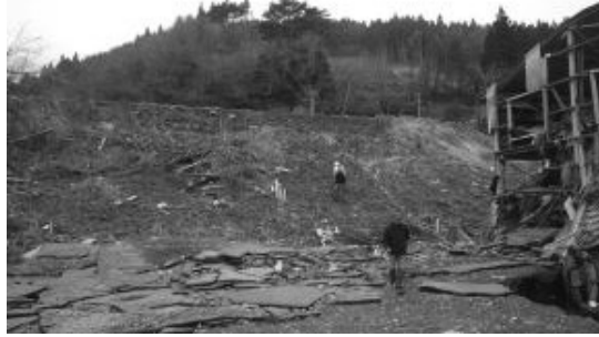
The tsunami ran over the 8m high railway embankment.
