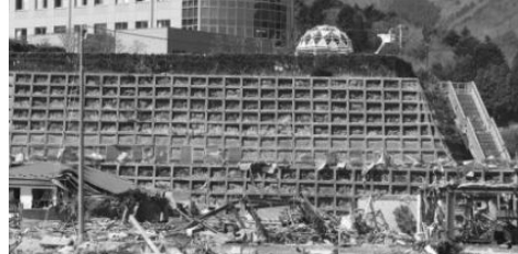
The tsunami reached the top of the wall.
