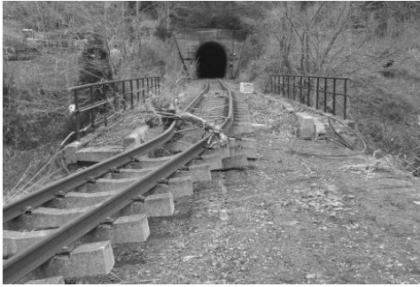
Rias line was shifted by the tsunami. The rails fell down from the embankment.
