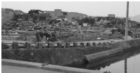
Large area of fire damage due to the tsunami
