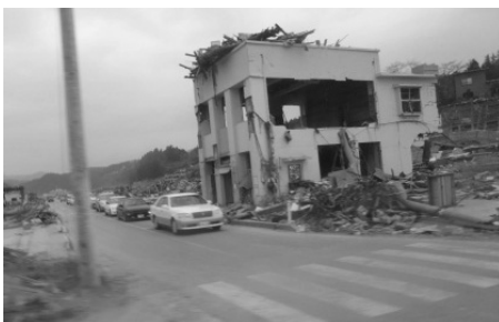
Damaged RC structure
