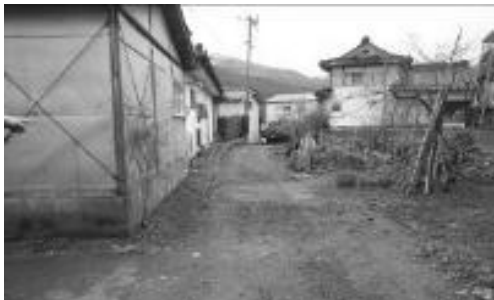
The tsunami swept behind the house.
