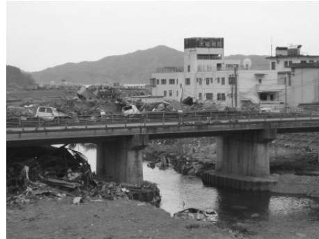
Damage to Otsuchi hospital
