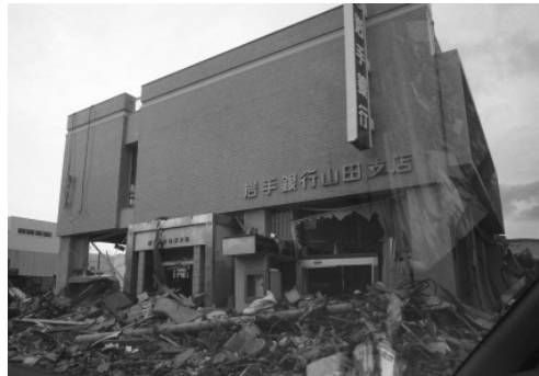
Damage to the Bank of Iwate, Yamada branch
