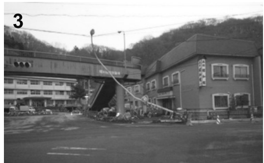
Broken pole in the front of the Showa-kan
