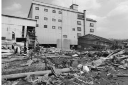
No major damage to the RC structure can be seen.
