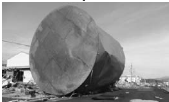
An industrial tank was overturned.
