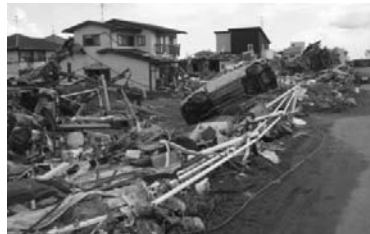
Damage area along the Nanakitagawa River, including fire damage
