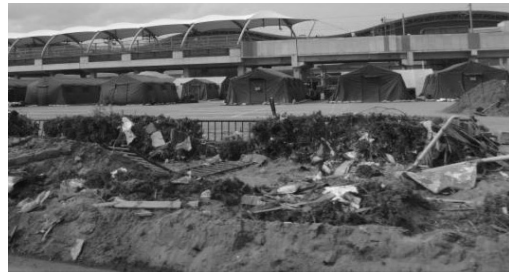
Damage to Sendai airport and the tents of the Self-Defense Force
