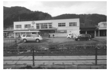
The extensive damage did not reach Kamaishi station.
