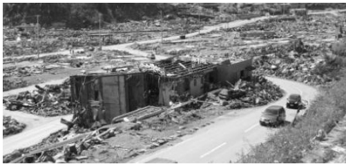
View of damaged town
