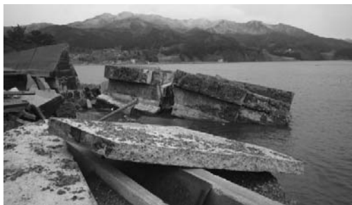
An embankment destroyed by tsunami.
