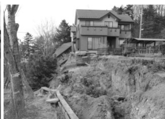
Houses damaged by slope failure; geotechnical damage was observed in housing development areas.
