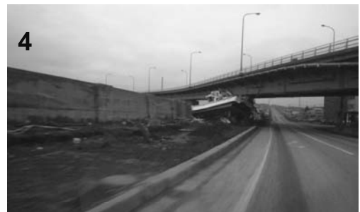
The boat shown here was swept up the Tsugaru Ishikawa from Miyako bay and stopped by the national road 45 bridge. The tsunami overflowed the river banks on the side of the Miyako city office building.
