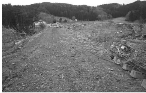
Rias line was shifted by the tsunami. The rails fell down from the embankment.
