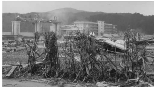
Sluice damaged by tsunami
