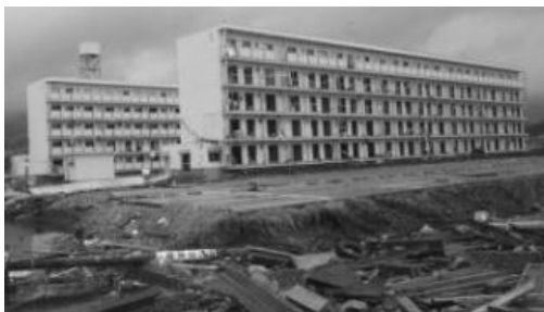
The tsunami reached up to the 5th floor of the RC apartment building.
