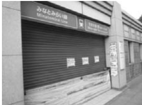
After the earthquake, all subway stations were closed (Nihonodori station, Yokohama city).
