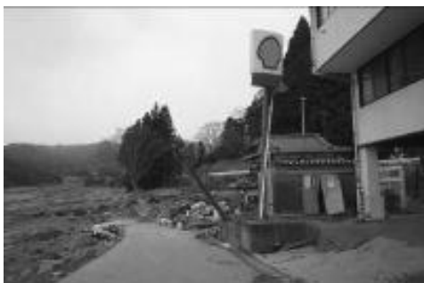
The tsunami reached the first floor of the gas station.
