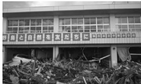
Damage to Nakano elementary school, located 1.2 kilometers from coast
