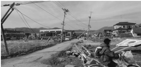
Bent poles and left over debris
