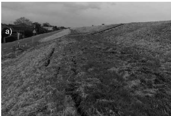
Photo 5. a) Cracking of Tone river dike in Kawachi Town, Ibaraki prefecture (site N) and b) sand boiling at its toe
