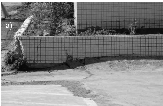
Photo 2. Boiled sand a) at reclaimed old swamp in Katori city, Chiba prefecture (site L) and b) at reclaimed old pond in Abiko city, Chiba prefecture (sites A and B)
