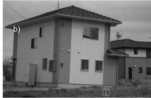
Photo 4. a) Tilt of wooden houses and failure of wall in reclaimed land of Urayasu city, Chiba prefecture (site RR) and b) tilt of wooden house at reclaimed old swamp in Itako city, Ibaraki prefecture (site LL)
