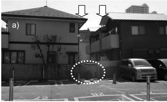
Photo 4. a) Tilt of wooden houses and failure of wall in reclaimed land of Urayasu city, Chiba prefecture (site RR) and b) tilt of wooden house at reclaimed old swamp in Itako city, Ibaraki prefecture (site LL)
