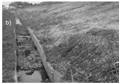
Photo 3. Boiling of gravelly soil at toes of Kokai river dike in Chikusei city, Ibaraki Prefecture (site Z)
