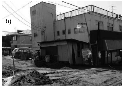
Photo 2. Boiled sand a) at reclaimed old swamp in Katori city, Chiba prefecture (site L) and b) at reclaimed old pond in Abiko city, Chiba prefecture (sites A and B)
