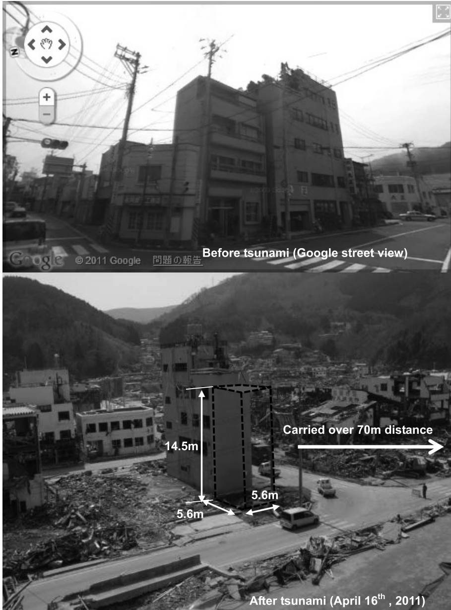
Figure 3 Original location of Building #1 (38.442482, 141.445728): This 4-story building was carried over 70m distance to the west.
