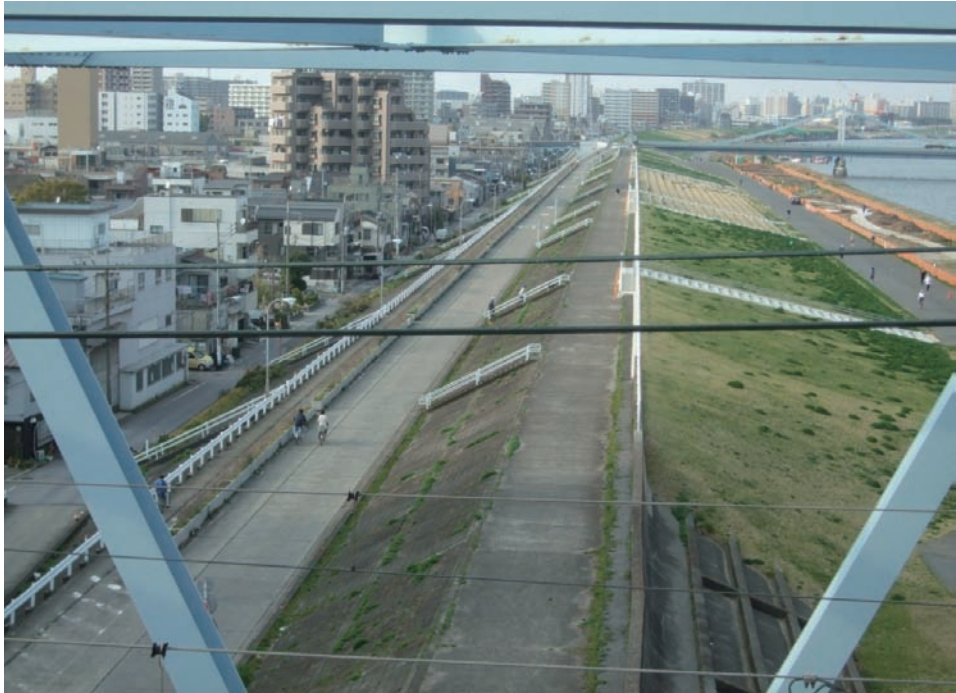
Figure 3(a) Upstream view of low-lying area near Arakawa Bridge of the subway Tozai line (35.665856,139.842868, Location is shown in Fig. 2): The area has been suffering from a serious land subsidence problem.
