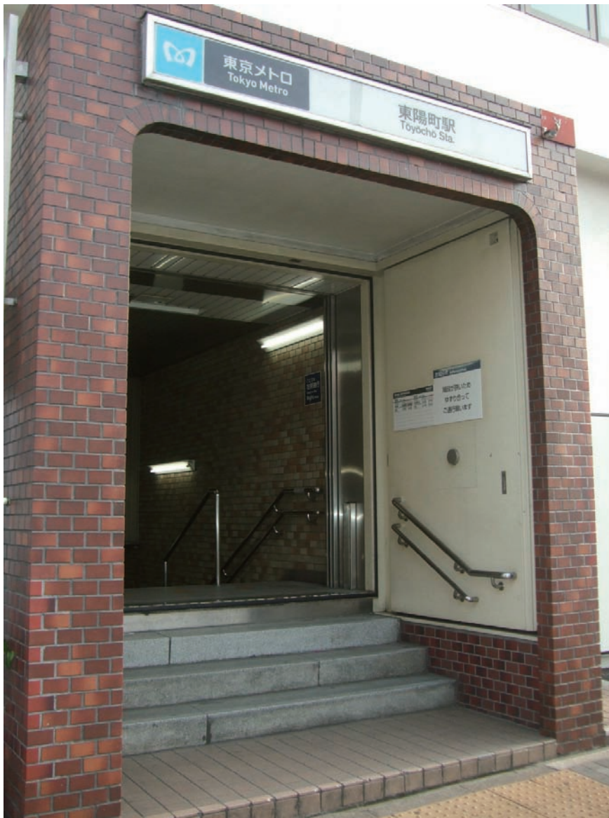
Fig. 4(b) Raised entrance of Toyochō Subway Station at 35.669469,139.816766: The entrance has a watertight door.
