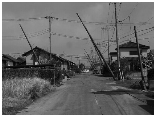
Photo 6 Damage of electric poles in Itako city
