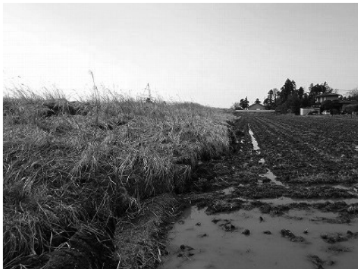
N38 32.223 E140 53.233 Photo 12 Levee suffered from lateral spreading (Naruse River)
