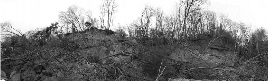
Photo 23 Slope failure occurred due to aftershock in Iwaki city
