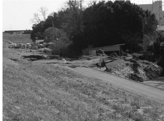
Photo 15 Liquefaction-induced damage of levee (Edogawa River)
