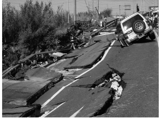
Photo 8 Damage of road by Liquefaction and tsunami in Kamisu city
