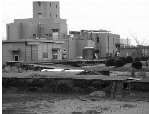
Photo 9 Liquefaction-induced damage of Wanigawa water treatment plant in Kamisu city
