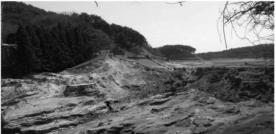
Photo 25 Breaching failure of Fujinuma earth dam in Sukagawa city
