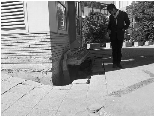
Photo 3 Differential settlement due to liquefaction in Urayasu city
