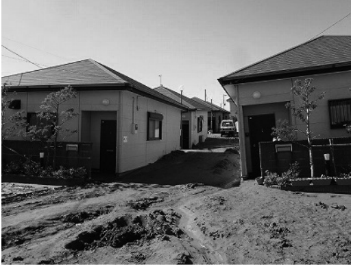
Photo 7 Uneven settlement of houses in Kamisu city
