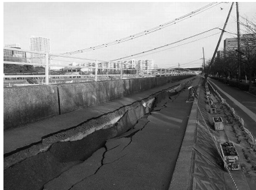
Photo 4 Settlement of backfill of retaining wall along Sakai River in Urayasu city
