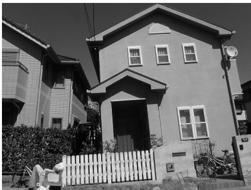
Photo 5 Uneven settlement of house due to liquefaction in Urayasu city
