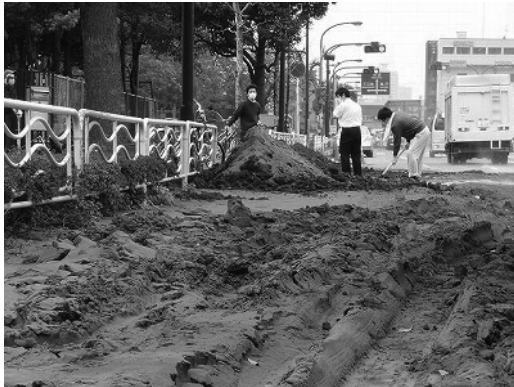
Photo 1 Boiled sand on the street in Shin-Kiba area
