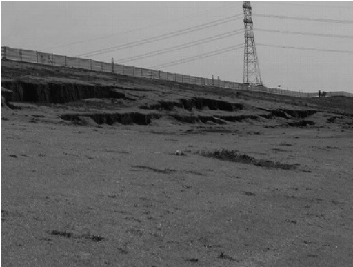
Photo 14 Liquefaction-induced damage of levee (Edogawa River)
