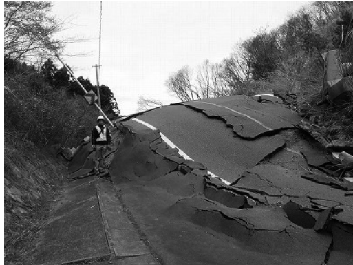
Photo 24 The failure of Photo 22 caused the foot of slope to uplift significantly.
