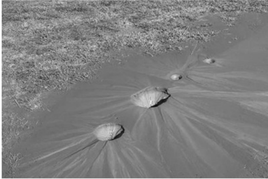
Photo 6 Boiled sand (Site 7 in Fig. 6)
