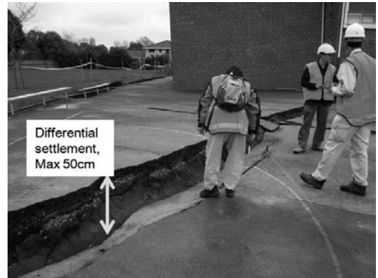
Photo 9 Pavement around St Paul's church suffered from large cracking and settlement (Site 26 in Fig. 6)
