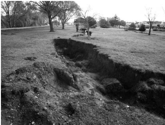
Photo 14 Significant cracking and boiled sand could be observed on the levee (Site 110 in Fig. 15)
