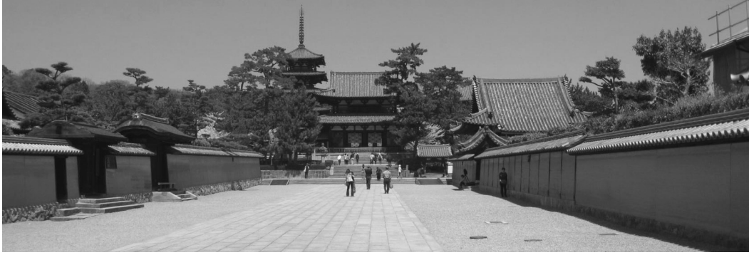
Figure 1. Rammed earth wall surrounding Horyu-ji temple, Hyogo Prefecture, Japan
