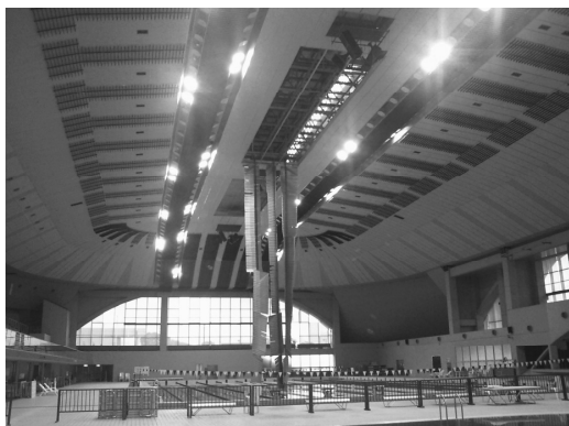
Figure 3. Public Pool-1 – hung louvers in the arena
