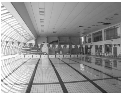
(a) Internal view
