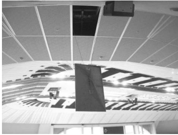
(a) Panel hung by an electric cable
