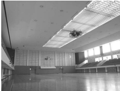
(a) Interior view
