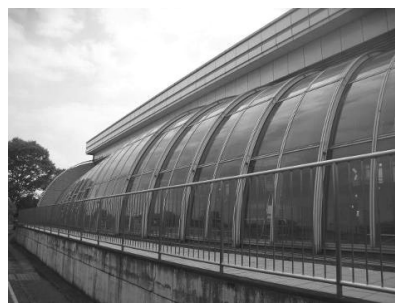
(b) External view (eastern side)
