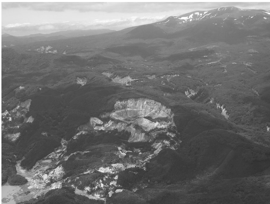
Fig. 7. Landslide mass behind the reservoir of Aratozawa dam (Photo by Konagai, K., June 15, 2008)
