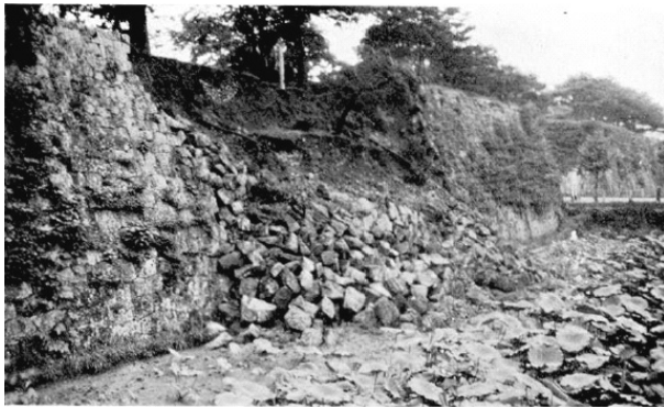
Fig. 2. Broken stone wall (No. 1 in the map below)
