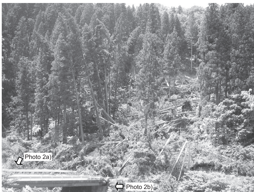
Photo 1. Slope failure at west side of Kurotaki bridge along prefectural road No. 51 (site A in Figure 2)
