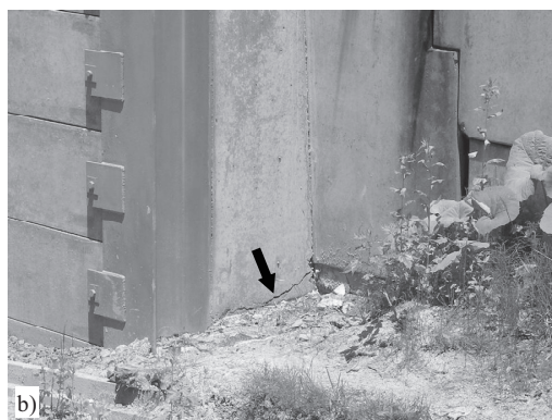
Photo 6. a) Reinforcement of approach embankment for Tochinoki bridge and adjacent reinforced soil retaining wall, b) Crack in reinforcement concrete beam of approach embankment
