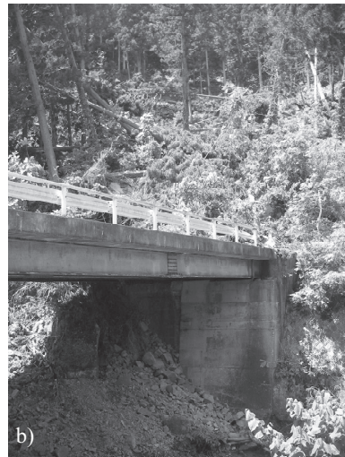
Photo 2. a) River course closure of Takamatsu river due to collapsed soil b) Abutment of Kurotaki bridge on the side of slope failure
