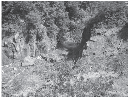
Photo 12. River course closure at Iwai river due to slope failure in Photo 11
