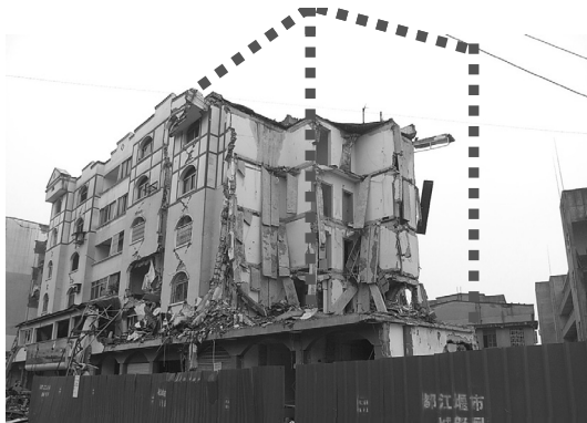
Photo 2. Partially collapsed brick buildings with precast concrete hollow-core slabs (Dujiangyan city)
