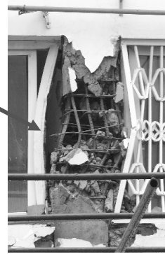
Photo 5. Shear failure in RC column shortened by partial height brick wall
