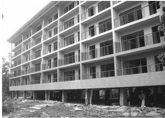
Photo 10. Example six story RC apartment building (See also Photos 6 and 7)
