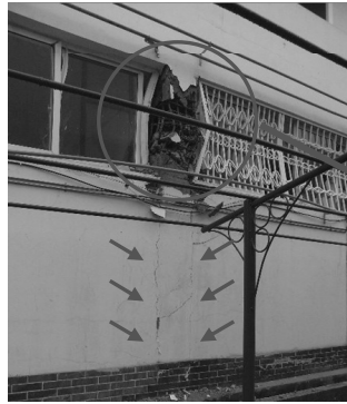
Photo 5. Shear failure in RC column shortened by partial height brick wall
