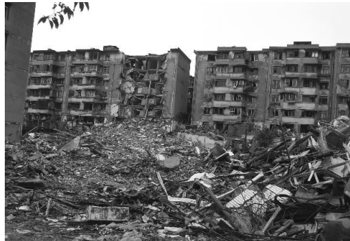
Photo 1. Seriously damaged brick buildings (Hanwang town of Mianzhu city)
