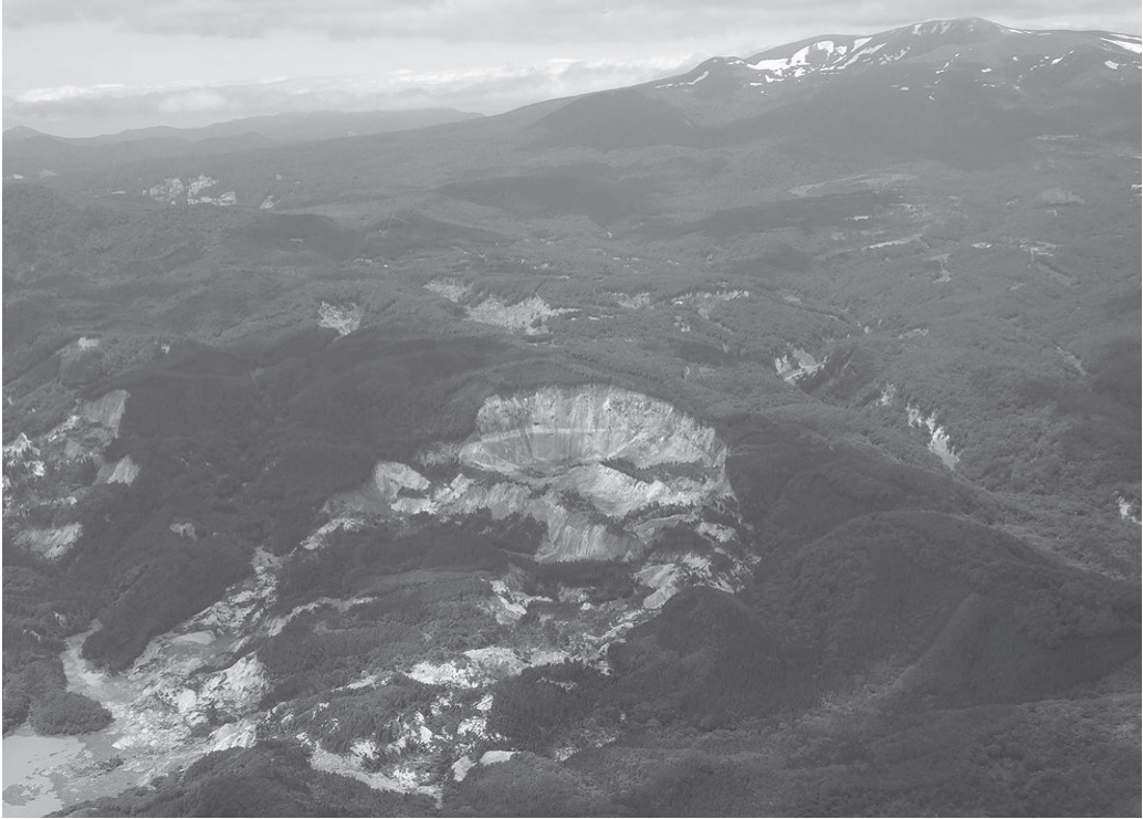
Fig. 1. Landslide at Aratosawa dam: (Photo by K. Konagai, June 15, 2008)
