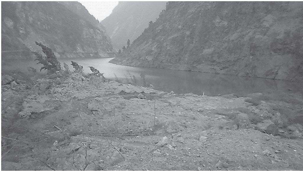
Photo 5. Landslide mass at “ShiBan-Gou” (Slate-Valley in English): (Photo taken on July 28, 2008, at 32° 25'55.5"N, 105° 06'32.2"E: Location estimated from Google earth: See Fig. 3)
