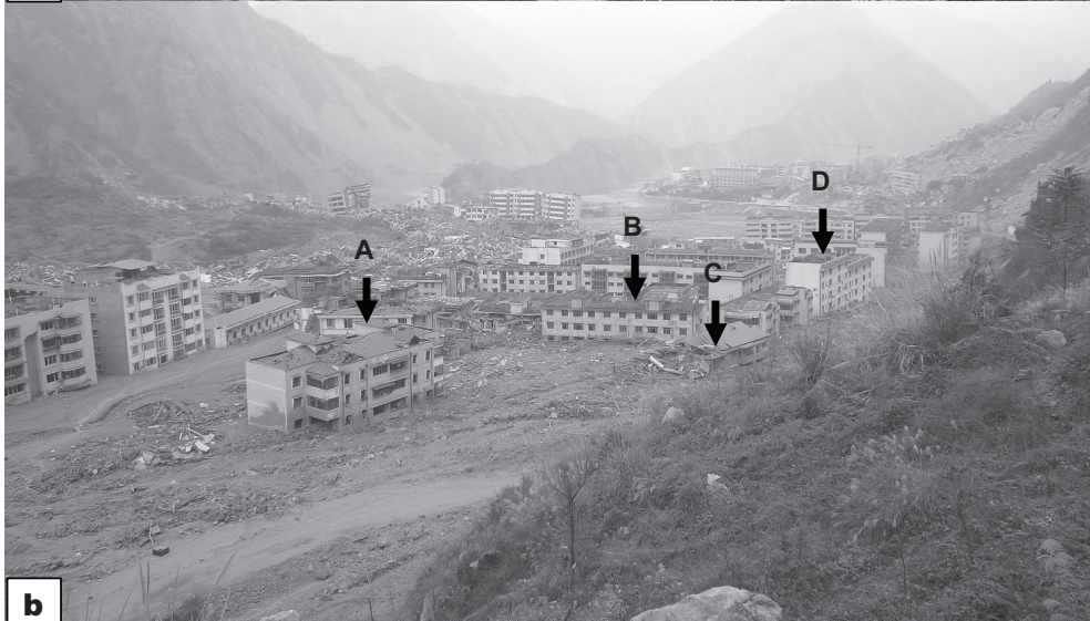
Photos 2a and 2b. South built-up area of Beichuan County. Photo 2a was taken on July 27 th , 2008 while Photo 2b shows the same area in December, 2008, buried beneath thick debris mass. (Photo 2b by Maki, N., DPRI, Kyoto University)
