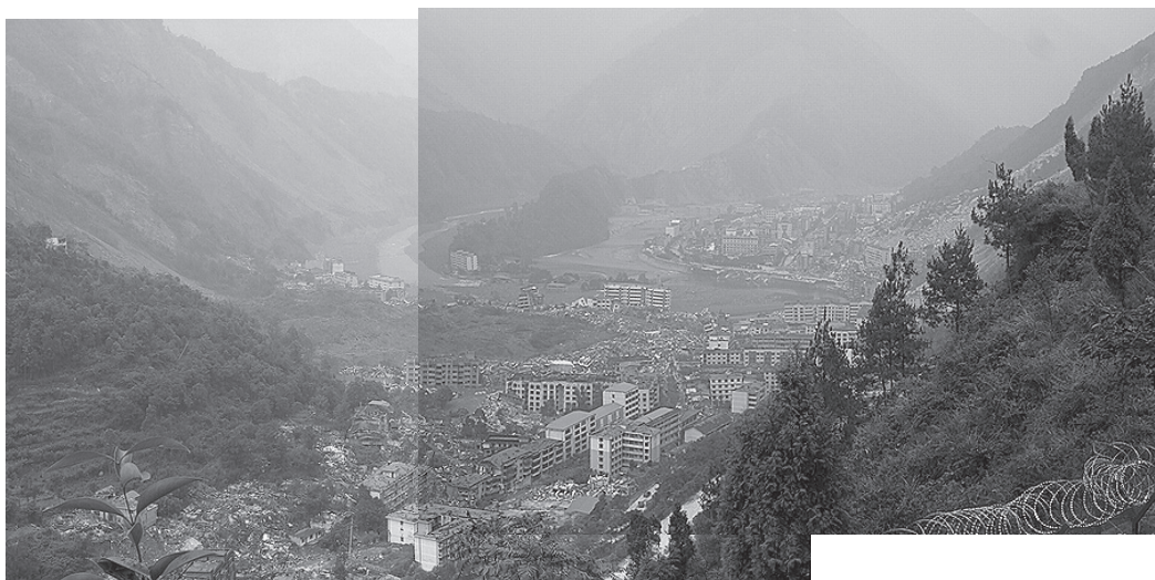
Photo 1. Downtown of Beichuan County. Two major built-up areas were completely destroyed by two major slope failures.
