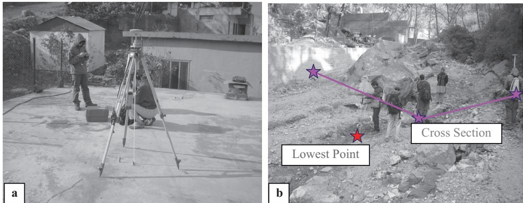
**Fig. 4:** GPS measurements along Gulshan and Tariqabad nallahs **a)** fixed reference station at roof of DAM office **b)** measurement for lowest point and cross section
