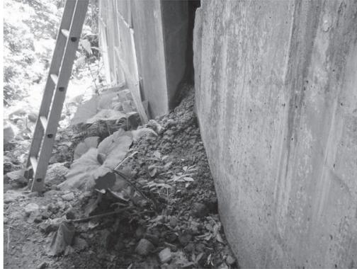
**Photo 7.** Outflow of backfill soil between reinforcement frame and original wing of Tochinoki bridge
