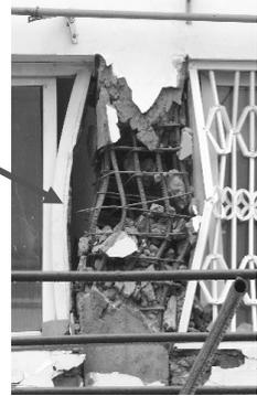
flexural compression failure at the top and bottom of their columns. Photos 6 and 7 show the damage to columns in the first story of a six story apartment building in Dujiangyan city. Hooks of lateral reinforcement are pulled out of crushed concrete core. Main rebars buckle and fracture as shown in the photos. As will be found later in this paper, the building is employed for a sample building to investigate possible restoration schemes and to discuss their feasibility with Chinese engineers.
