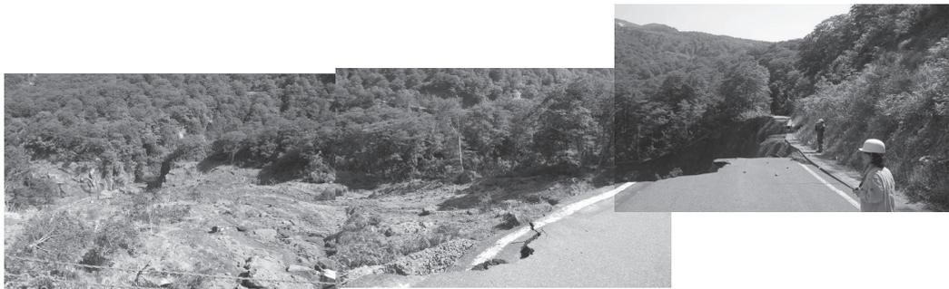
**Photo 11.** Large slope failure including embankment along National Highway route No. 342 (site D in Figure 2)
