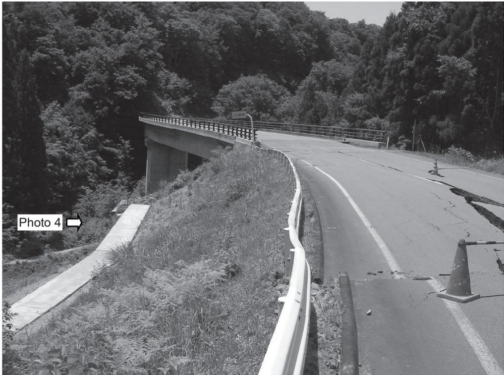
**Photo 3.** Settlement of approach embankment for Shirakaba bridge along national highway route No. 398 (site B in Figure 2)
