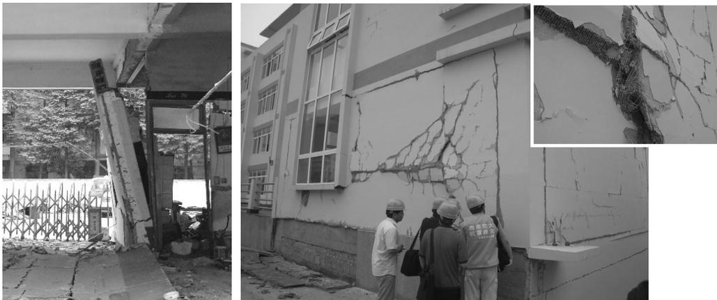
**Photo 3** Failed brick wall (left) and survived brick wall (right)
