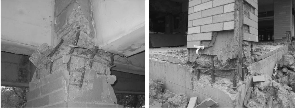
**Photo 7.** Flexural compression failure at the top and bottom of columns
