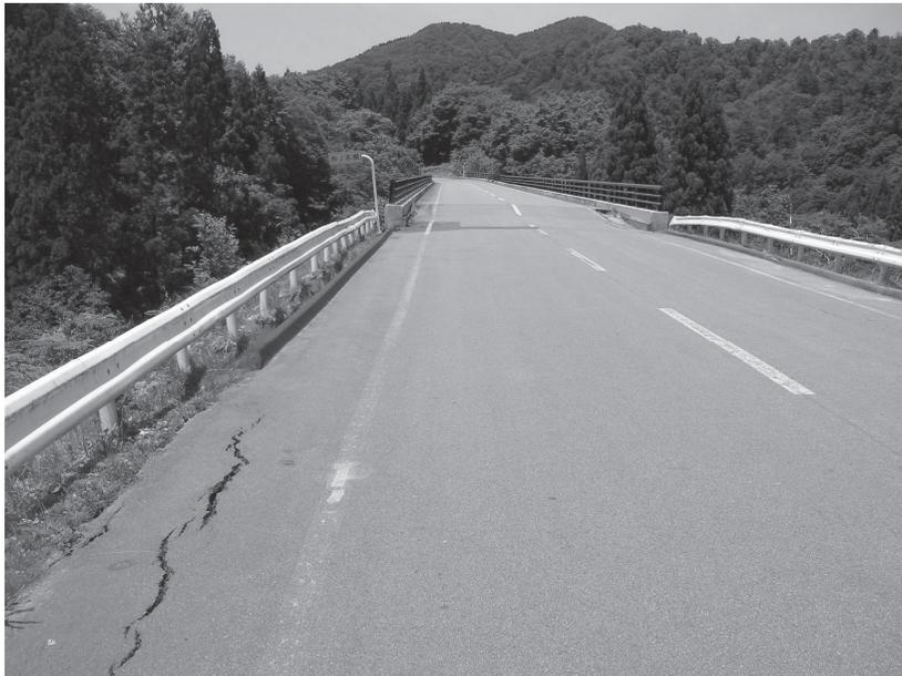
**Photo 5.** Settlement of approach embankment for Tochinoki bridge along national highway route No. 398 (site B in Figure 2)
