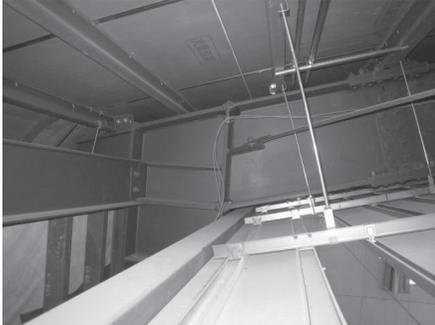
**Figure 20.** Hunger bolts normal to the slope near edge-line of ceiling at Gymnasium-5
