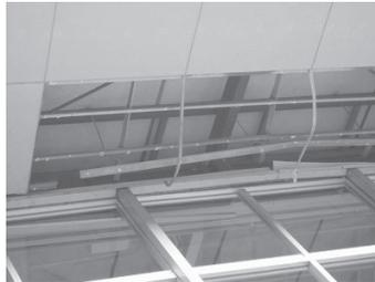
(b) Deformation of runner under exterior eave
