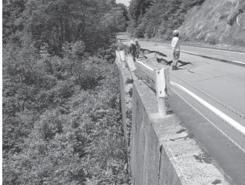
**Photo 9.** Tilting and settlement of gravity type retaining wall in Photo 8
