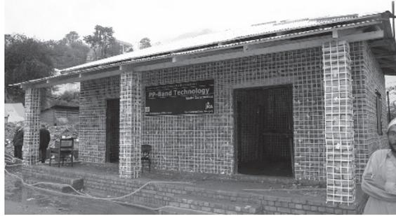
**Figure 2.** PP-band retrofitted house before mortar laying
