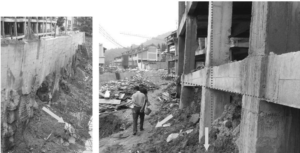
**Photo 9.** Structural damage due to failure in retaining wall
