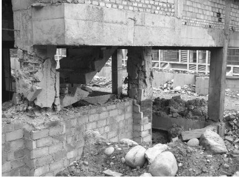
**Photo 4.** Typical shear failure in RC short columns
