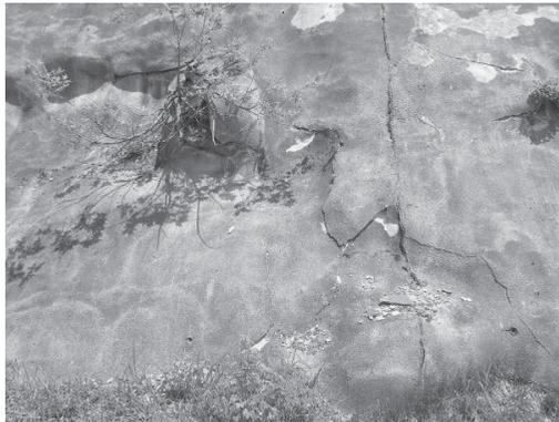
**Photo 10.** Cracks in shotcrete on cut slope
