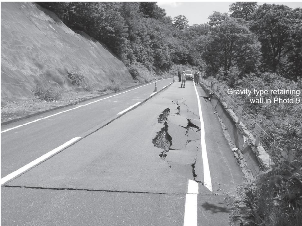
**Photo 8.** Collapse of embankment along national highway route No. 398 (site C in Figure 2)
