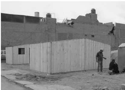
Figure 25. Wooden temporary house
