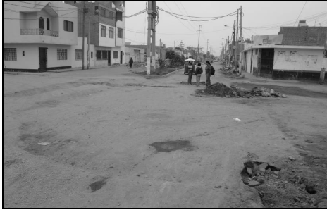
Figure 8. Central Pisco. Settled ground as evidence of broken sewer pipes.
