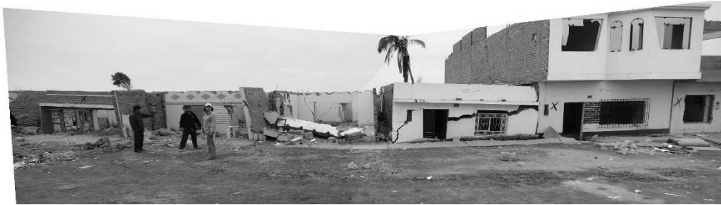
Figure 5. Settlement of 0.7 m of building in front of palm tree.
