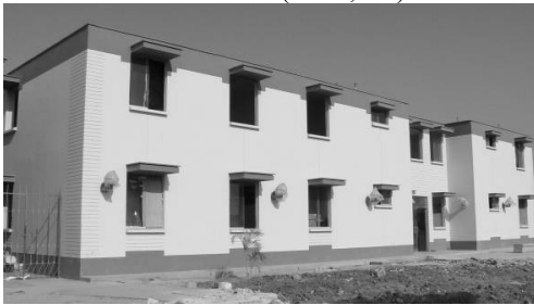
Figure 16. New Emergency Building suffered no damage (San Juan de Dios Hospital)
