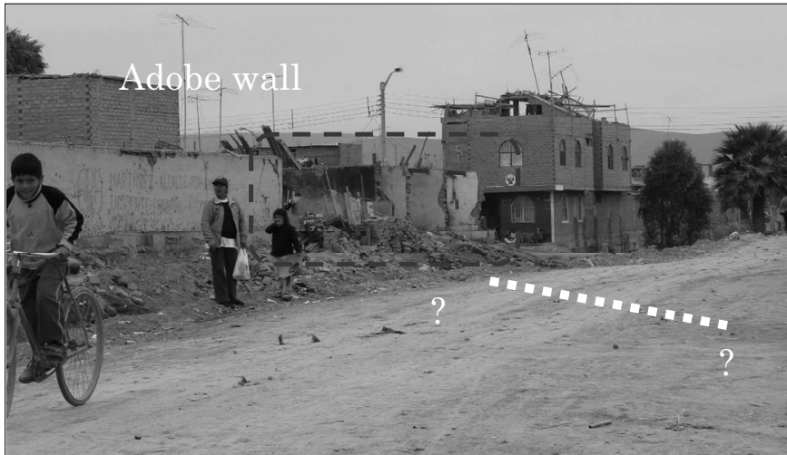
Figure 11. Collapsed adobe house due to large ground cracks in Nuevo Monterrico. The local people told us the crack crossed the street. The adobe wall to the left did not collapse.
