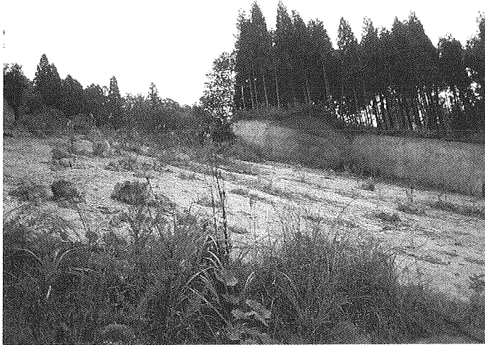
Figure 1. Slope failure investigated in this study
