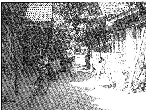
Photo 12. Houses condition at Site H
