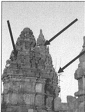
Photo 33. Damage to Prambanan temple at Site X
