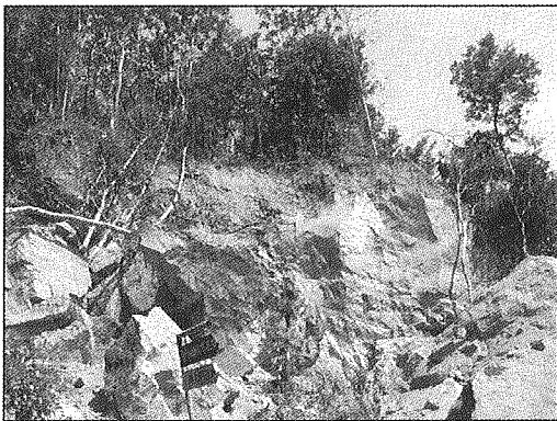
Photo 25. Rock fall at Site R
