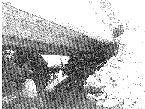
(c) Four simple beams support the deck.
