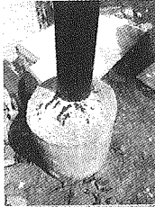
Fig. 1. No clear cracking of lamp post pedestal was found. (Pesu, Klaten)
