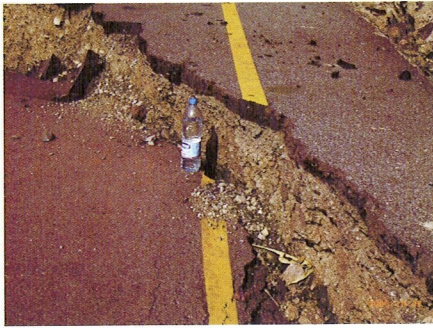
Fig. 34: Road No. 6, north of Balakot (Site C in Fig. 36)
