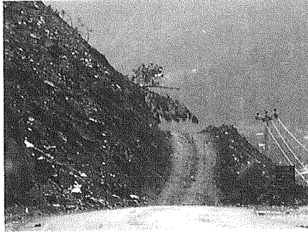
Fig. 18: Road No.6, Site No. 14
