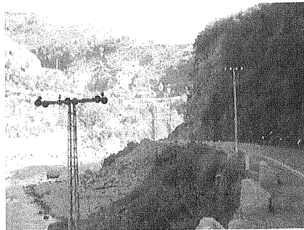
Fig. 11: Road No.3, Site No. 7
