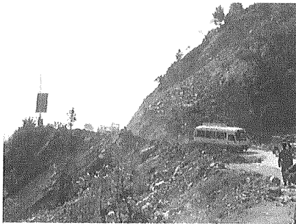
Fig. 14: Road No.5, Site No. 10
