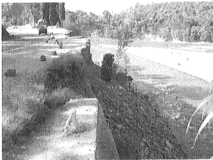
Fig. 26: Road No. 3, east of Muzaffarabad
