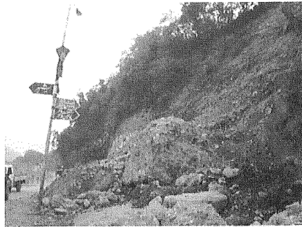
Fig. 5(a): Road No.1, Site No. 2
