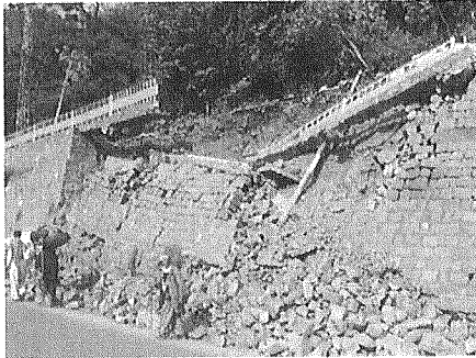
Fig. 24: Local road in Muzaffarabad
