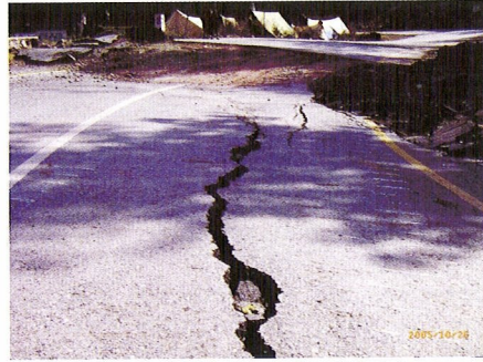
Fig. 35: Road No. 6, north of Balakot (Site D in Fig. 36)
