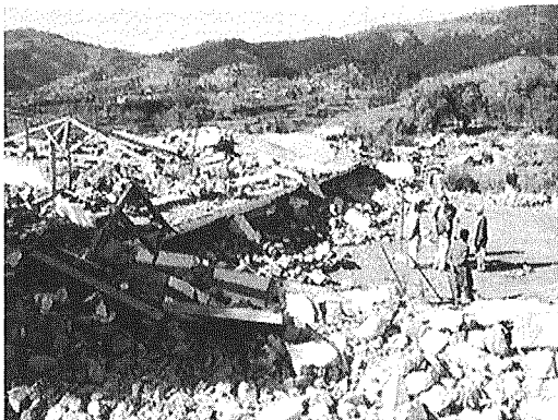
Photo7-1. Collapsed primary school
