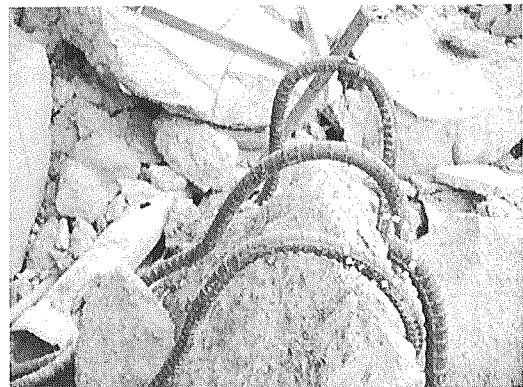
Photo 11-4. Fractured rebar
