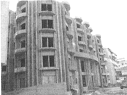
Photo 4-1. General view of Al-Safa Heights
