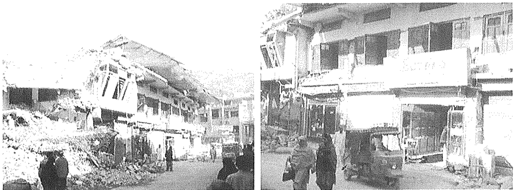
Photo 13-4. Continuously occupied vulnerable buildings
