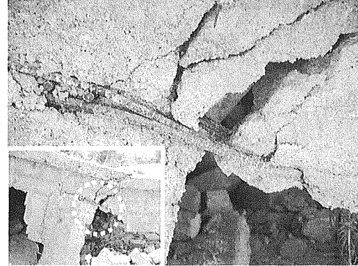
Photo 12-3. Beam rebars outside reinforcement cage
