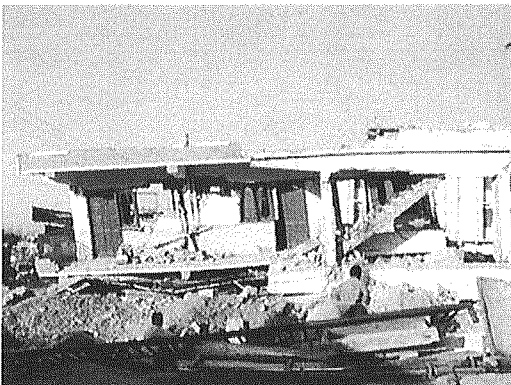
Photo 10-1. General view of collapsed restaurant
