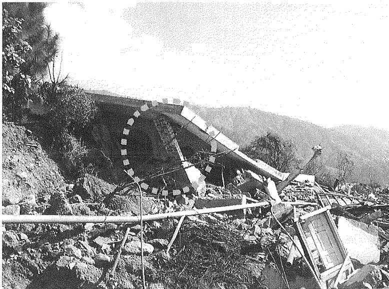
Fig. 9. Foundation and column of a dwelling at the long-bean-shaped hill
