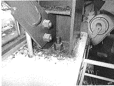
(c) No damage to the structural elements
