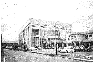
(a) Exterior view
