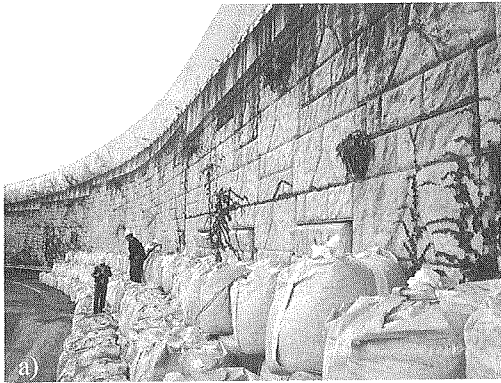
Figure 8. Damage to a retaining wall reinforced with metal strips and its temporary rehabilitation along JH Kan-etsu Expressway (at Horinouchi Parking Area; site 5 in Figure 1)
