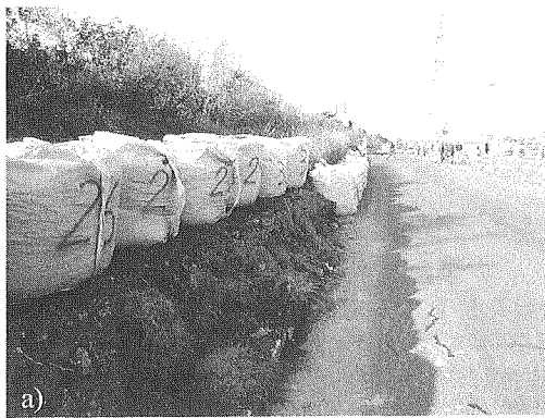
Figure 9. Damage to an embankment along JH Kan-etsu Expressway and an adjacent regional road (at Sakura-machi, Ojiya city; site 6 in Figure 1)
