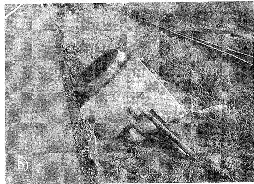
Figure 21. Complete uplift of buried pipes and tilting of an uplifted manhole along National Highway Route 117 (at Yachi, Ojiya city; site 14 in Figure 1)
