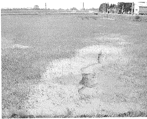
Figure 19. Sand boils on ground behind a dike along the Shinano river (at Iwano, Koshiji-machi; site 12 in Figure 1)
