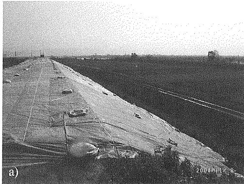
Figure 16. Temporarily rehabilitated dike along the Shinano river and a sand boil on adjacent ground (at Namiki-shinden, Nakanoshima-machi; site 10 in Figure 1)
