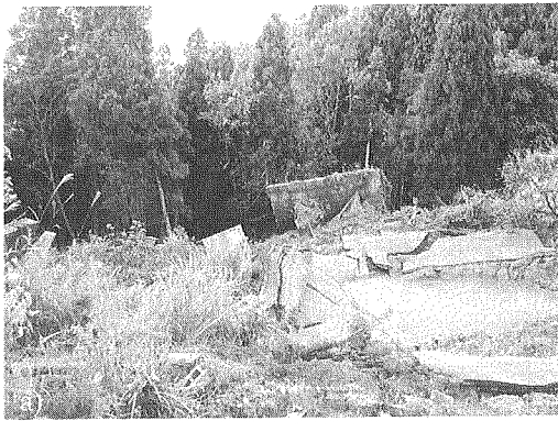
Figure 12. Collapse of an embankment for regional road around newly-developed building estates (at Taka-machi 3-chome, Nagaoka city; site 7 in Figure 1)
