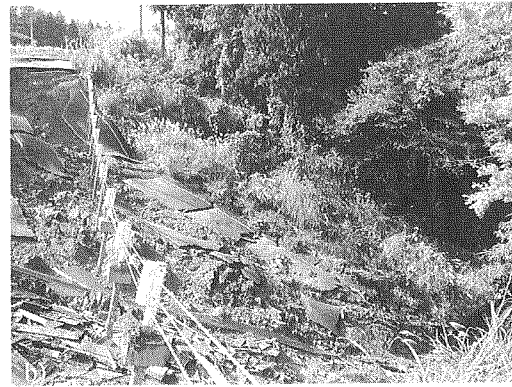
Figure 7. Collapsed embankments along National Highway Route 290 (at Kuriyama-zawa, Tochio city; site 4 in Figure 1)
