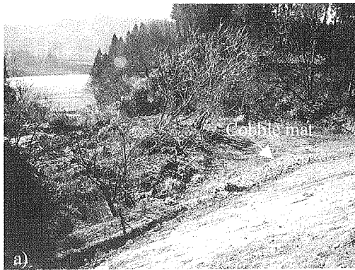
Figure 3. Reconstructed embankment and reinforced soil retaining wall along JR Joetsu line (site 1 in Figure 1)
