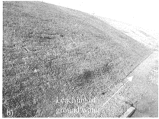
Figure 14. Damage to a dike along the Shinano river (at Chiya-gawa, Ojiya city; site 8 in Figure 1)
