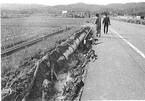
Figure 21. Complete uplift of buried pipes and tilting of an uplifted manhole along National Highway Route 117 (at Yachi, Ojiya city; site 14 in Figure 1)
