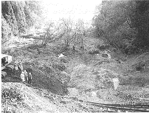
Figure 2. Collapse of an embankment along JR Joetsu line (between Echigo-Kawaguchi and Ojiya stations; at Hiu, Ojiya city; site 1 in Figure 1)
