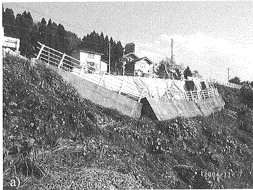
Figure 5. Damage to a retaining wall along National Highway Route 17 and an adjacent embankment along JR Joetsu line (at Kamikatagai, Ojiya city; site 3 in Figure 1)
