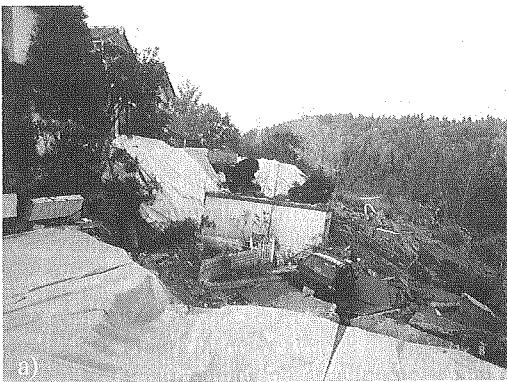
Figure 13. Collapse of an embankment for regional road around newly-developed building estates (at Taka-machi 1-chome, Nagaoka city; site 7 in Figure 1)
