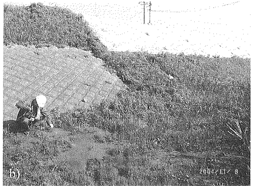
Figure 16. Temporarily rehabilitated dike along the Shinano river and a sand boil on adjacent ground (at Namiki-shinden, Nakanoshima-machi; site 10 in Figure 1)
