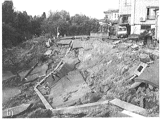
Figure 12. Collapse of an embankment for regional road around newly-developed building estates (at Taka-machi 3-chome, Nagaoka city; site 7 in Figure 1)
