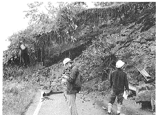
(b) Landslide #2 in Fig. 4
