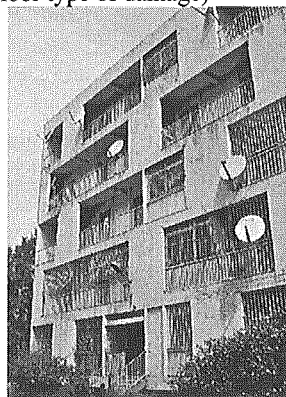
(c) Structure 3 (5-story RC building)
