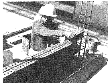
Figure 5. Horizontal reinforcement anchored to the vertical confinement.
