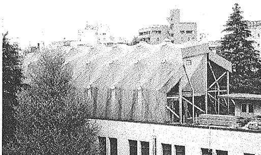
Photo 1: Tension truss dome (Model as a whole with membrane)
