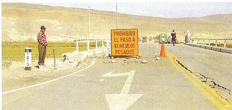
Figure 18: Settlement of bridge approach and cracking of road. Only one lane is open for traffic (looking in southbound direction).
