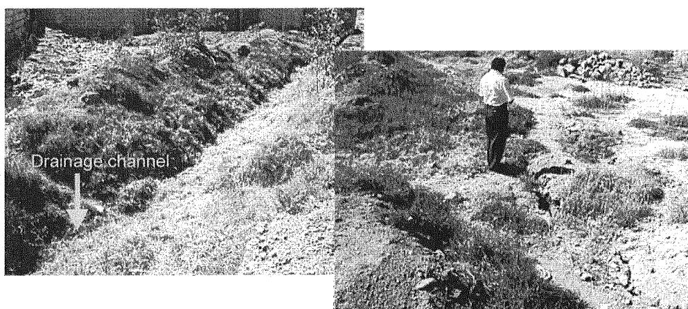
(a) Lateral spreading toward drainage channel
