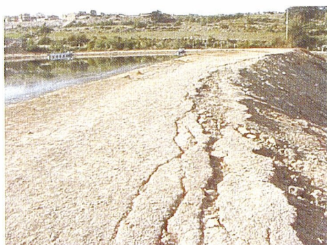
Figure 14. Longitudinal cracks
