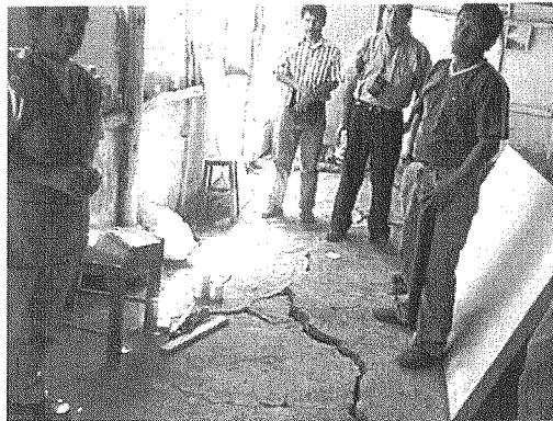
(e) Heave of house floor due to sand boil Figure 10 Liquefaction-related damage (continued)
