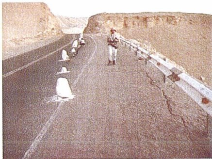
(a) Settlement of embankment crest
