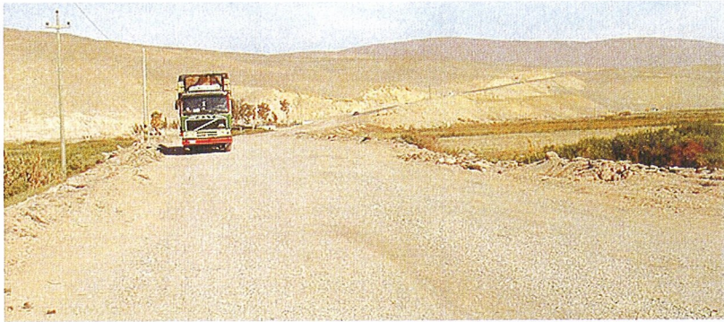
Figure 16: Pan American Highway Pavement removed after damaged due the earthquake (looking in Southbound direction).
