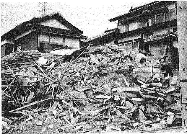
Fig. 8 Flattened house at Saihaku town:
