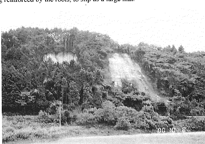
Fig. 5 Landslide at Furuichi
