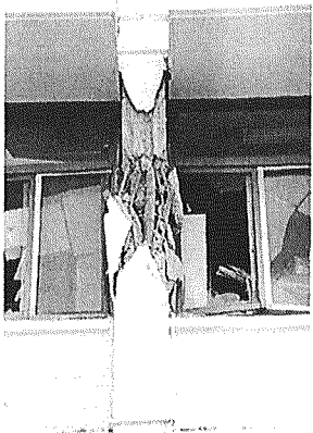
Figure 4: Damage Example Photos (left: RC columns / right: brick walls)
