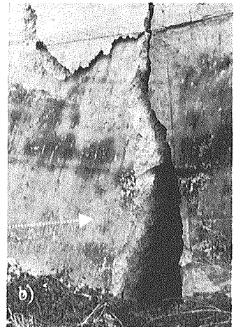
Plate 3. Damage to gravity type retaining wall due to failure of subsoil layers (along District Road No. 129; site 3 in Fig.1)
