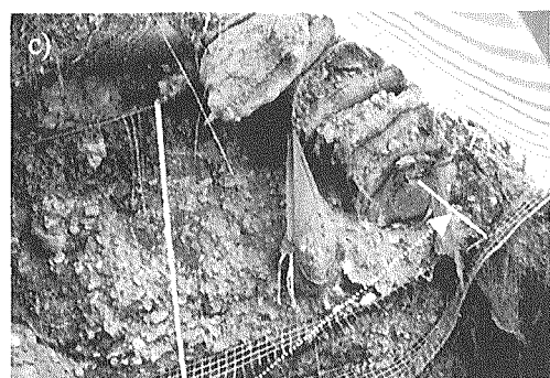
Plate 10. Damage to wrapped-around type reinforced-soil embankment (at National Chi-Nan University; site 8 in Fig. 1)
