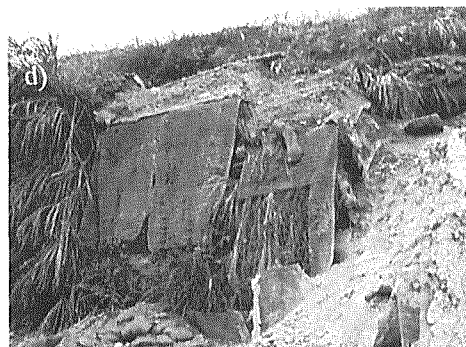
Plate 10. Damage to wrapped-around type reinforced-soil embankment (at National Chi-Nan University; site 8 in Fig. 1)
