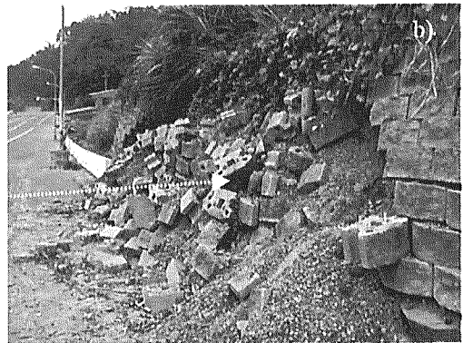
Plate 7. Damage to reinforced-soil retaining wall using keystones as a facing (along District Road No. 129; site 2 in Fig. 1)
