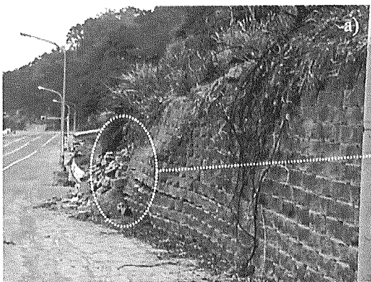
Plate 7. Damage to reinforced-soil retaining wall using keystones as a facing (along District Road No. 129; site 2 in Fig. 1)
